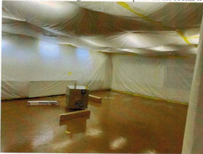
As room was being sealed for the asbestos removal
